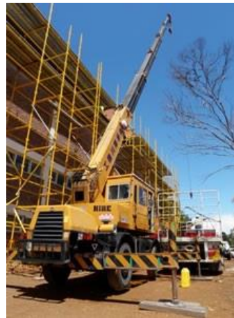
Typical single pole putlog scaffold
